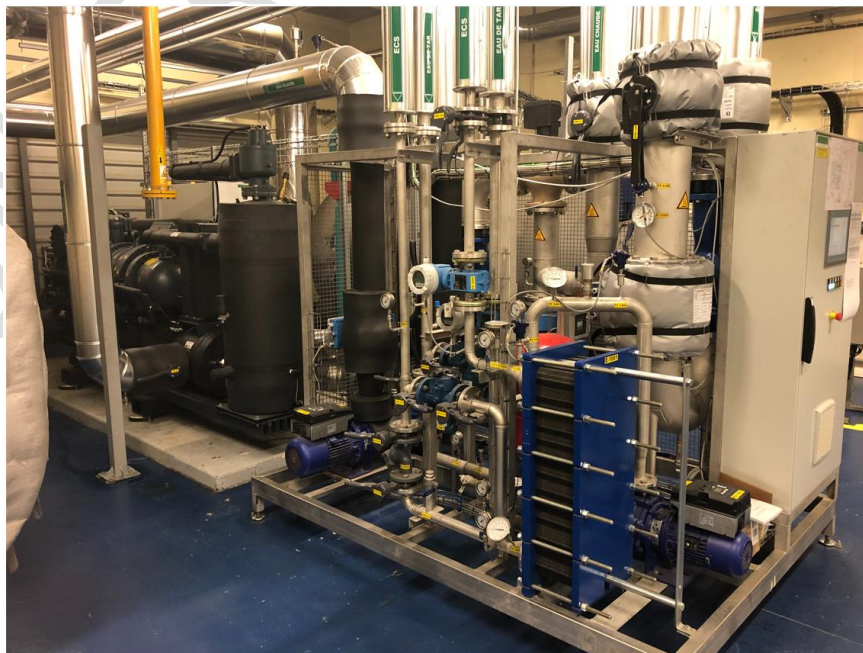
Figure 12. Rear view of the Heat pump & Production Skid
