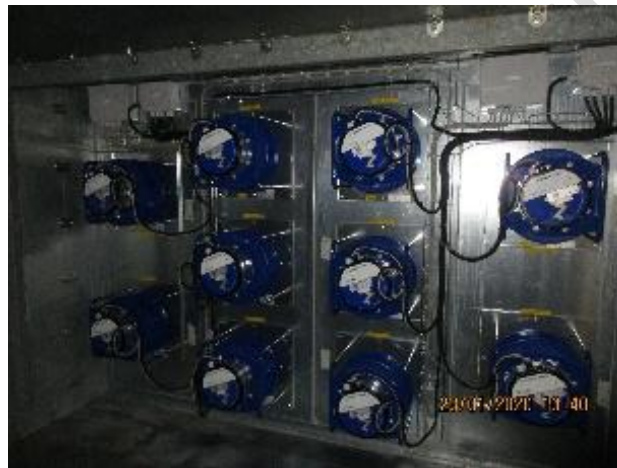
Figure 4. Direct drive multi grid fans with EC motors
