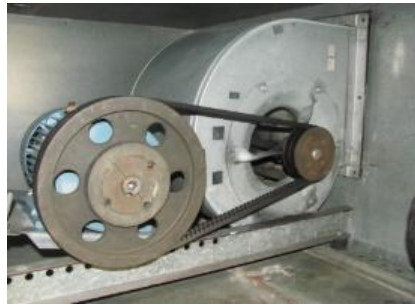
Figure 3. Belt drive fan with conventional motor
