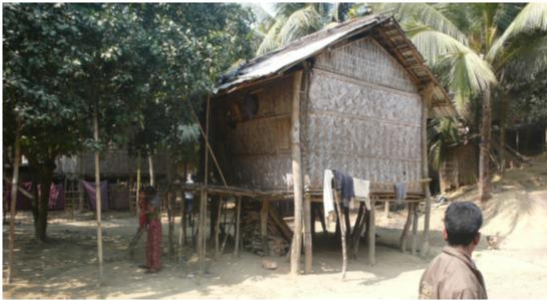
Figure 1: Flood resistant housing in Bangladesh [16]
