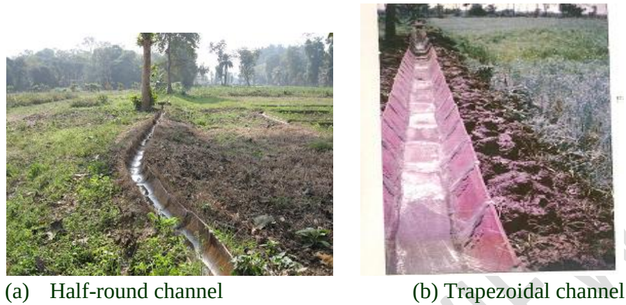
Fig. 6 Half-round and trapezoidal earthen tile made channels
