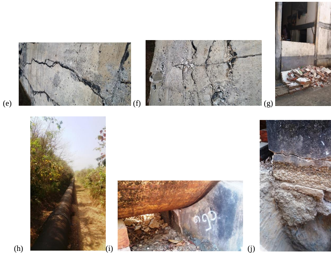
Fig.3.(a,b,c) Photos of damage to a building in which upper floor was fallen to the ground due to Taikkyi earthquake. (e,f) damage to the pavement of the road in Taikkyi. (g) Damage to the wall of a building. (h,i,j) Damages at the base of Gyophyu pipeline.
