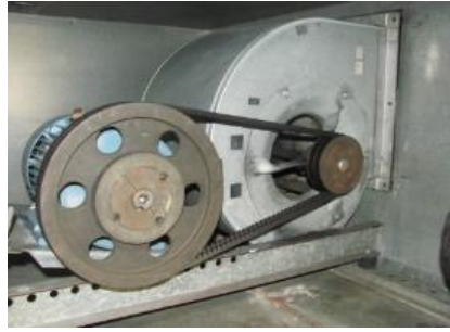
Figure 3. Belt drive fan with conventional motor
