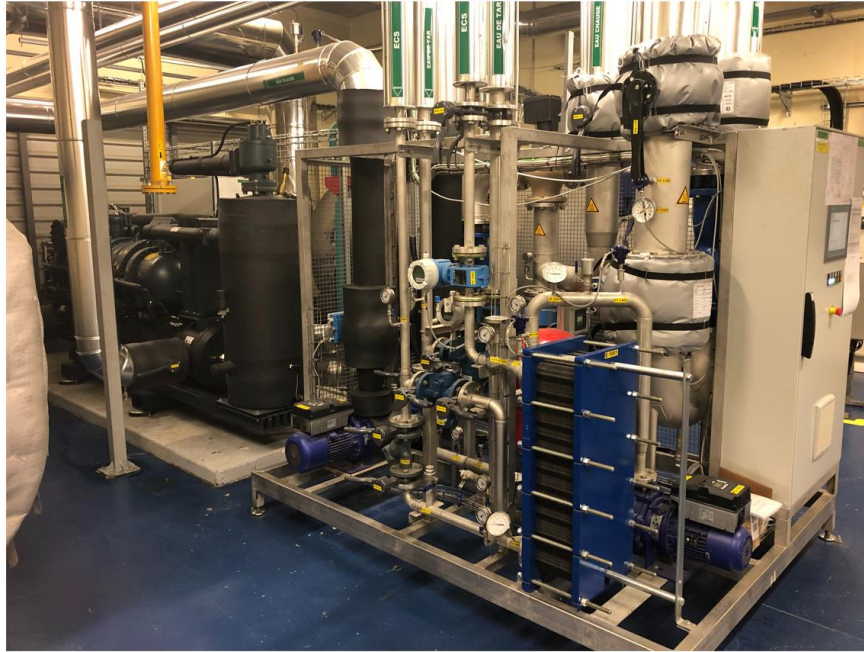
Figure 13. Rear view of the Heat pump & Production Skid
