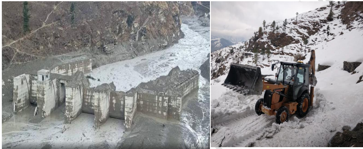
Fig 4 (a): Dhauliganga hydropower project affected breaking of glacier at Joshimath Feb. 7, 2021. Fig 4(b): The Avalanche riské area in Himachal Pradesh Feb'2019 The avalanche occur under conditions of snowstorm Strong western disturbance, when the overburden surpasses 200\text{kg}^2 after filling the terrain irregularities like Rishiganga and Dhauliganga power house project in the year 2021 (Fig 4(a) and Fig 4(b) (Singh et al, 1998; Podolsky 2010 [12] ).
