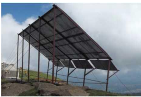
Fig 6(d): Jet roofs avalanche prone area
