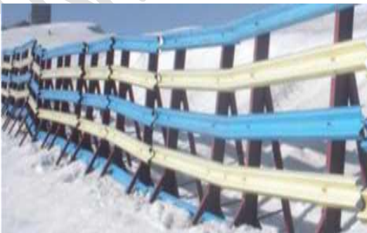
Fig 6(c) : Snow fences in avalanche area
