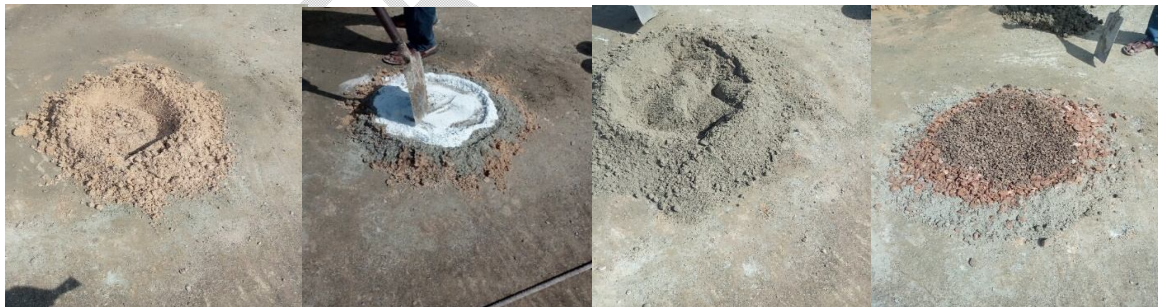
(d) Coarse aggregate and shells of palm kernel added to the mixture of cement, recycled glass powder and fine aggregate
