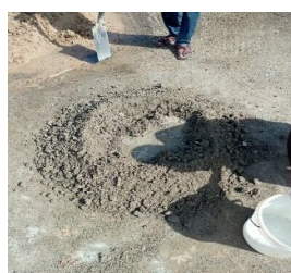
(e) Mixture of fine aggregate, cement, recycled glass
